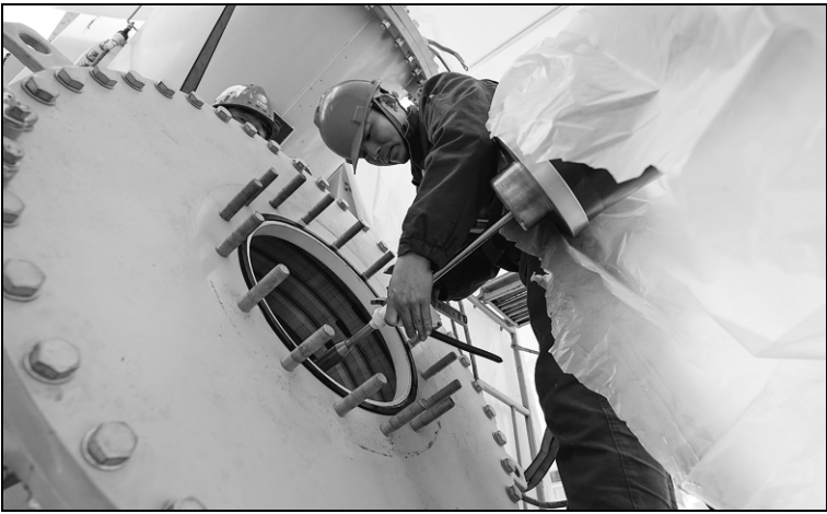
Right: A worker installs a spare rectifier transformer bushing at Balikun converter station in Hami, Xinjiang. DING LEI / XINHUA
