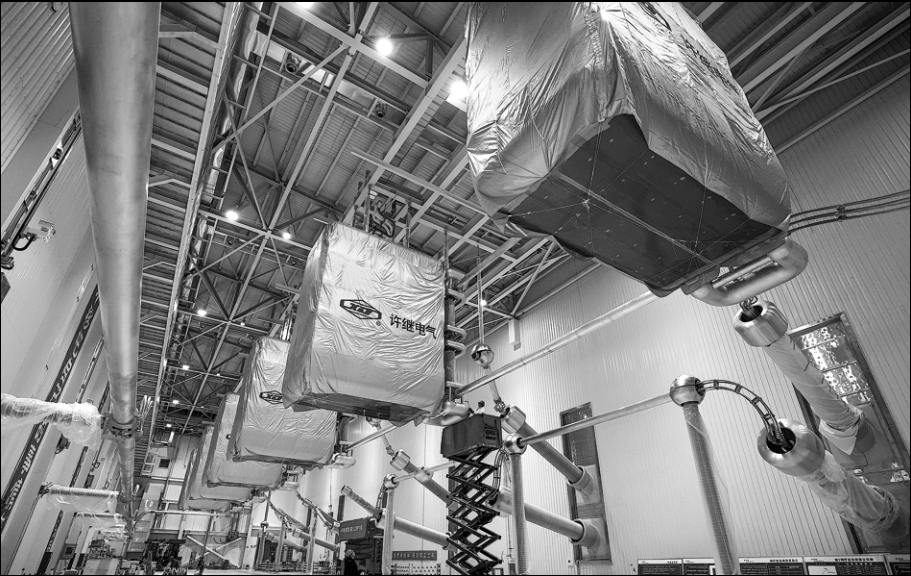
A technician inspects hardware in the valve hall of Balikun converter station in March. DING LEI / XINHUA
